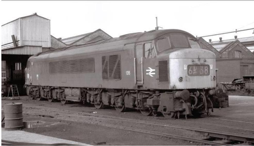
135 showing the modified headcode arrangement following repairs at Derby Works
